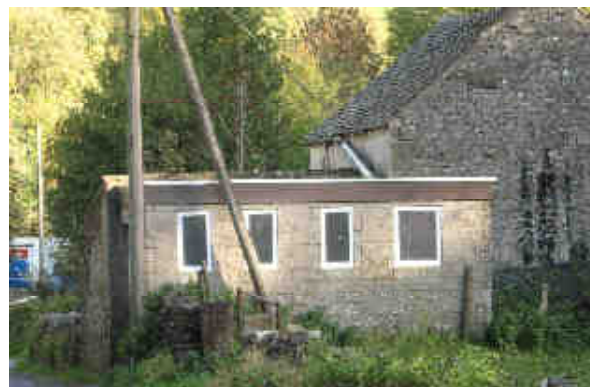
Flat roofed toilet block
