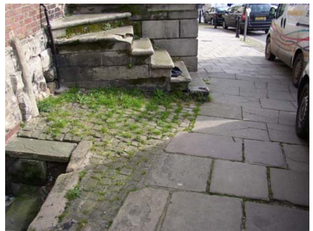
7. Yorkstone flags and sett detail corner of Buxton Road and King Street.
