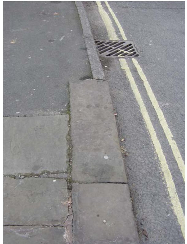
Detail of robust stone kerb detail on Buxton Road, alongside narrow concrete kerb and tarmac.
