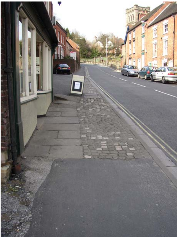
2. Mix of patchy tarmac, stone flags, stone setts and kerbs at southern end of Buxton Road (north).
