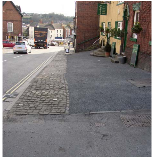
3. Tarmac area fronting 'Brambells' with some stone setts to road side (south).
