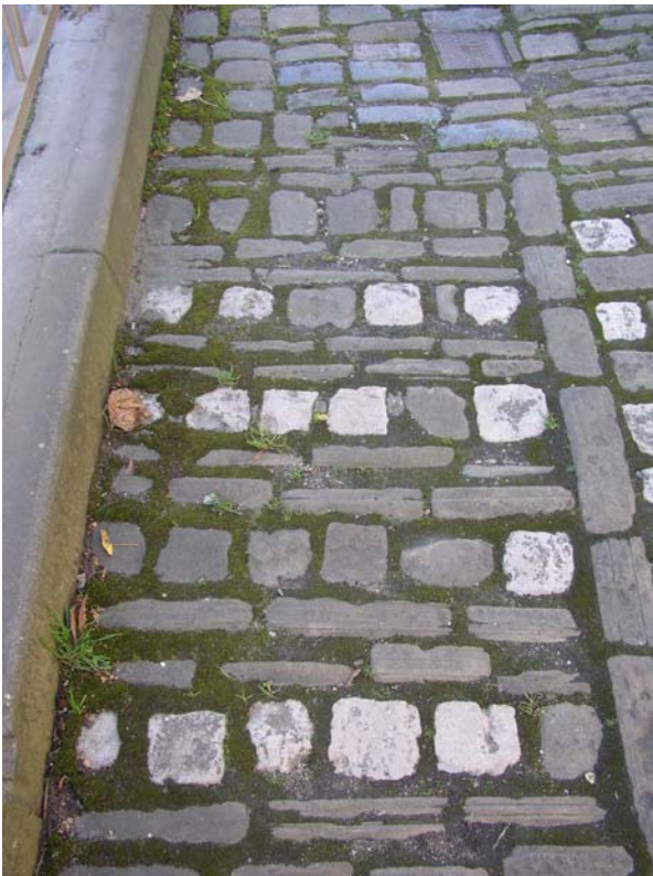
As above - Detail of pattern formed by the use of square limestone and gritstone setts alongside gritstone setts laid lengthways.
